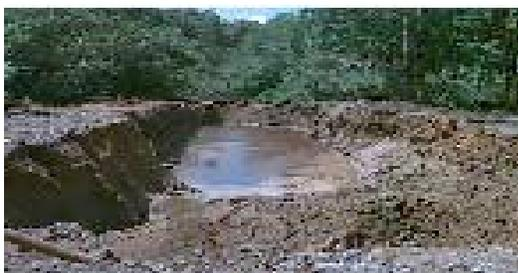
*Based on test results and RAB recommendations, Westover’s contractors excavated potentially contaminated areas behind the former Jet Test Stand due to concerns about contamination.\**
